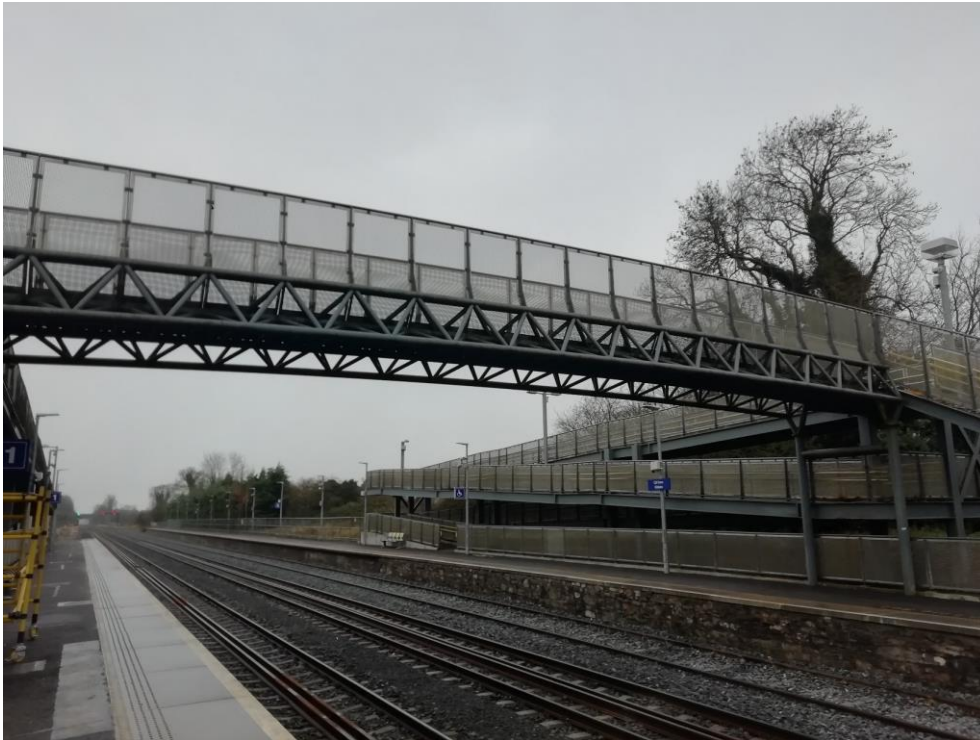
Figure 8.19: Existing Ramp Kildare Town Train Station
